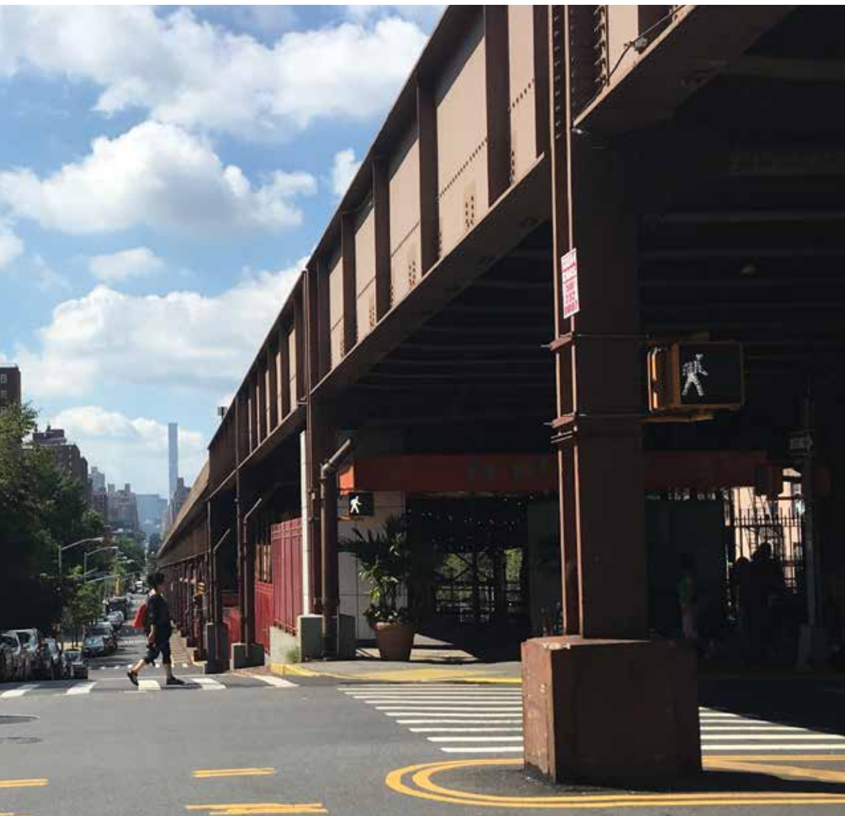
The East Harlem Neighborhood Plan aims to revitalize the blocks surrounding the elevated MetroNorth tracks with transit-oriented, high-density mixed uses.
